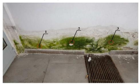
Photo 2. The three sampling points (marked 1,2,3) on the biodeteriorated external building wall
