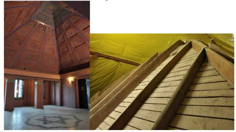
Fig. 5, 6. Mourning hall with a pyramid vault (following renovation) and wooden structure of the self-bearing vault [photograph by A. Skrzypińska, 2014]
