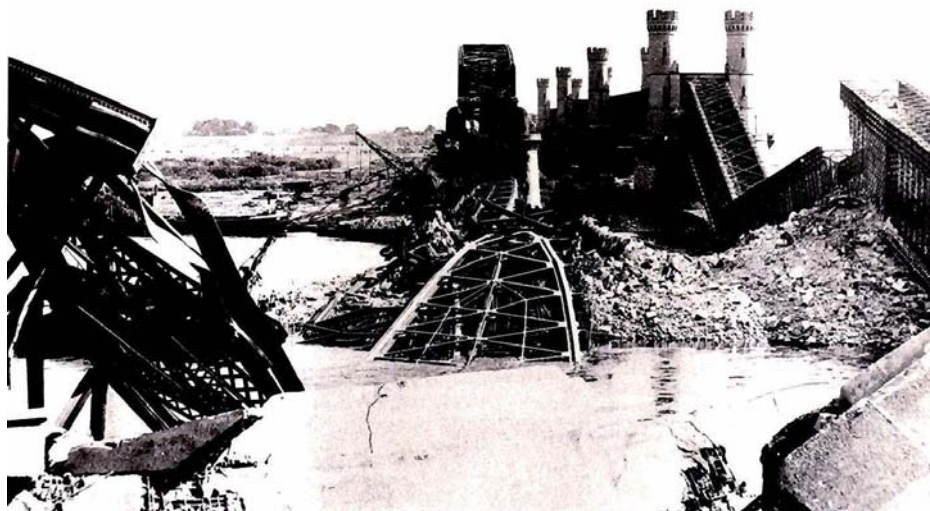
Fig. 3. War damages of bridges in 1938
