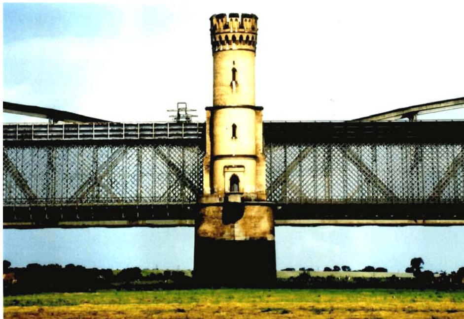
Fig. 5. Side view of bridges
