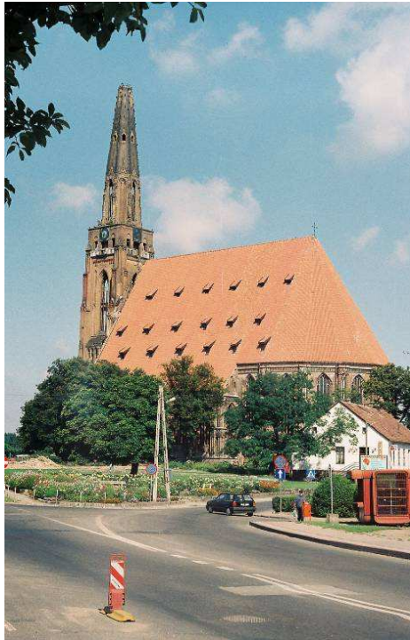
Fig. 7. Church at the end of the I stage of reconstruction; view from south-east
