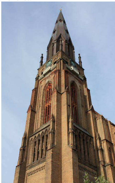
Fig. 9. Church after completion of II stage; photo by M. Płotkowiak
