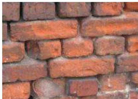
Fig. 4. The effects of corrosion in the wall on lime mortar of lower strength than brick
