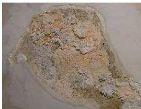
Fig. 2. Crystallization of the salt within the plaster
