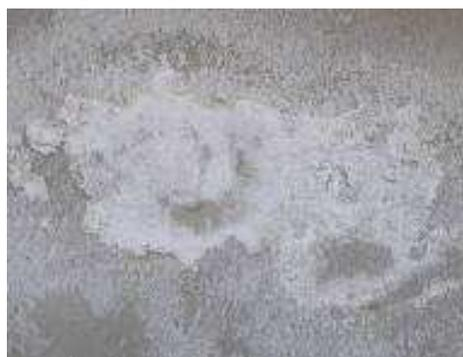
Fig. 1. Surface crystallization-wall and plaster remain overdamped
