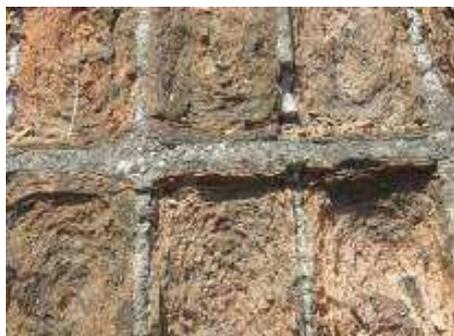
Fig. 3. Effects of corrosion with cement mortar stronger than ceramic material
