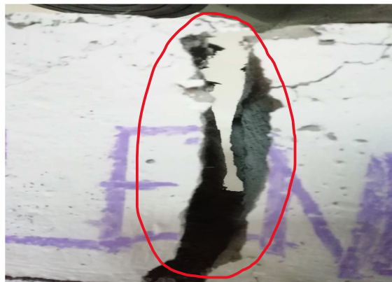
Fig.9. Failure of unreinforced CLC prism
