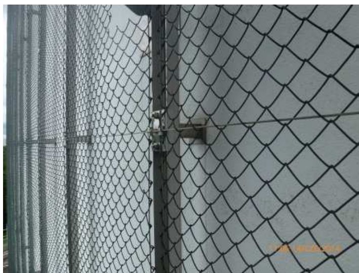
Fig. 6. Construction for green wall - Philharmonic Hall in Białystok
