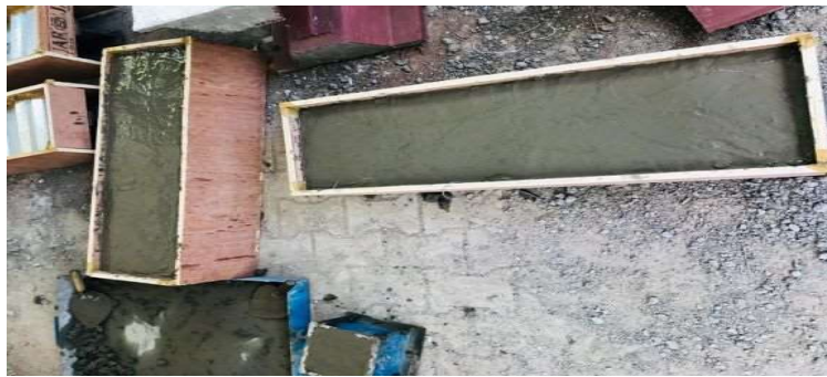
Fig. 3. Composite beam after placing of concrete
