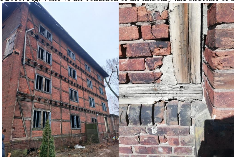
Fig. 4. Elevation of the retrofitted building, condition of the masonry samples author archive
