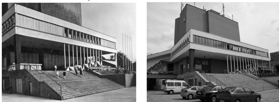
Fig. 9-10. The attitude of full acceptance – the theatre in Rybnik, designer J.Gottfried, H.Buszko and A.Franta, (1958-1964). State before and after modernisation in 2006 designed by J.Wawrzyniak. Full respect for the historical value of the object. The project included the preservation of a number of details such as the floors which retained their original form (i.e. broken slate floors) or Marian Rak's fresco adorning the entrance to the auditorium. Photo by R. Nakonieczny.
