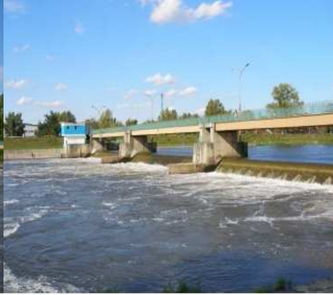
Fig. 4. Weir Opatowice – view from left bank
