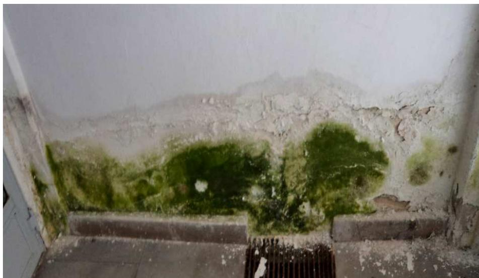
Photo 1. The external building wall with visible biocorrosion on the building of the former UZ canteen
