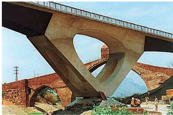
Fig. 5. A bridge of double composition with a prestressed concrete pier interacting with the bridge bottom plate in abutment section ("del Diabolo" bridge near Barcelona).
