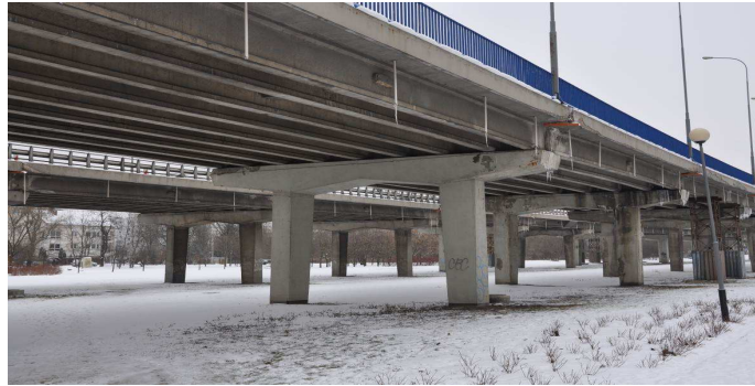
Fig. 3. Composite concrete-concrete bridge in WBS system (a flyover in Poznań).
