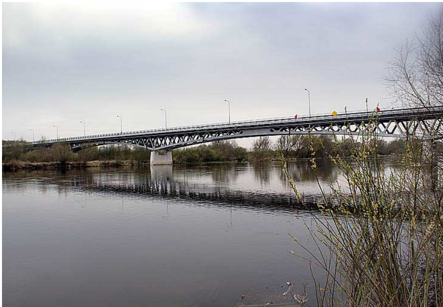
Fig. 1. Bridge over the Bug river in Brok (Poland)
