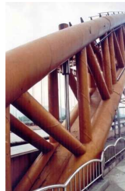
Fig. 29. Truss concrete filled steel tubular (CFST) through bridge of 200 m span, near Quilin (China)
