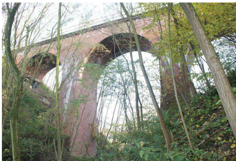
Fig. 4. General view of the bridge C
