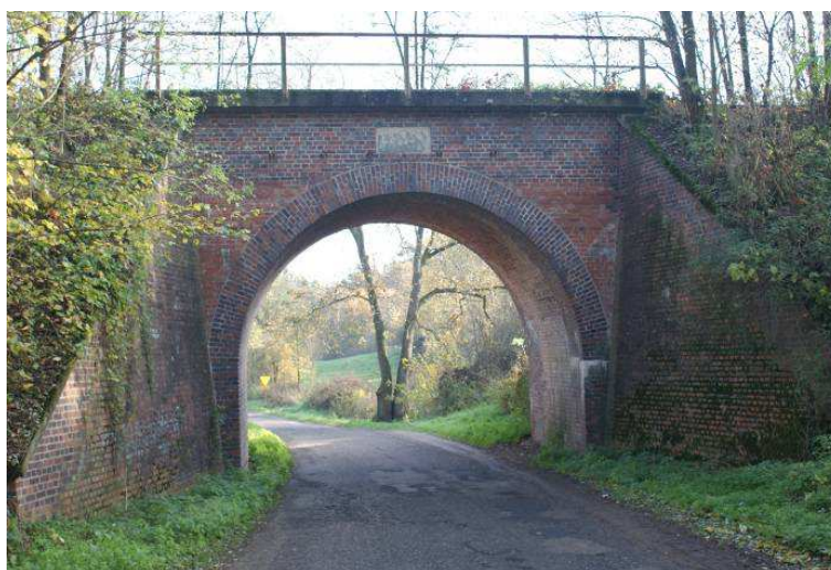
Fig. 5. General view of the bridge D
