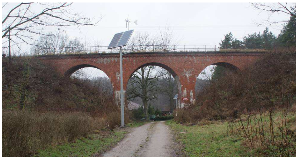
Rys. 3. General view of the viaduct B
