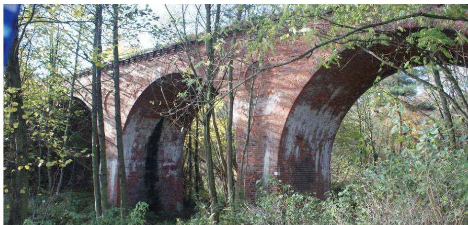
Fig. 2. General view of the bridge structure A
