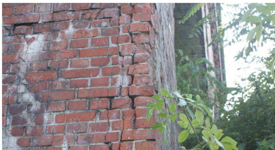
Fig. 7. View of viaduct pillar B. Visible cutting of the outer layer of bricks
