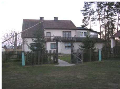
Fig. 1. Building on farm 1
