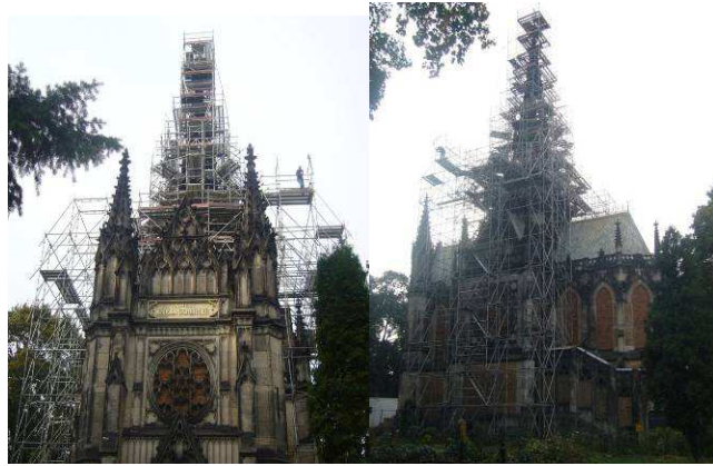
Fig. 3. Scaffolding around the Chapel of Scheibler
