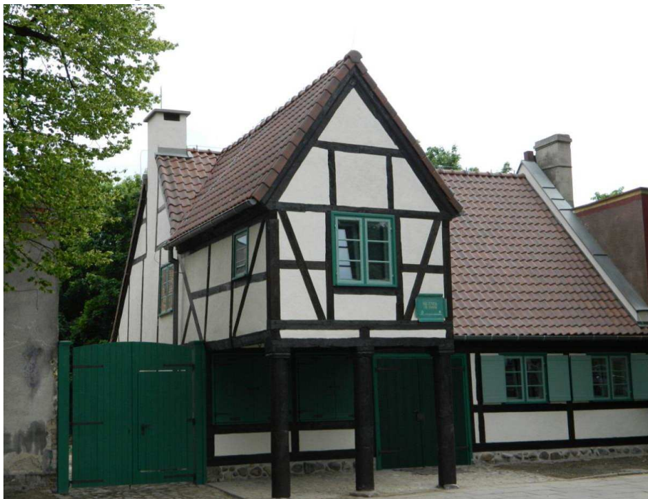
Fig. 1. Forge building after completion of construction-conservation work
