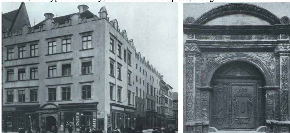
Fig. 1a, 1b. Building "Zur goldenen Krone" and its portal by the end of XIX c
