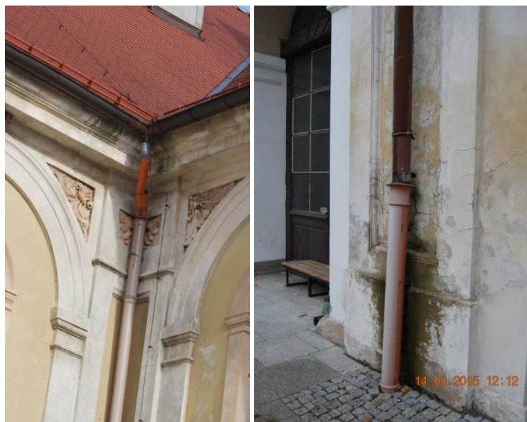
Fig. 12, 13. Existing connections of the downspouts on the east façade (fot. W. Sokołowski)
