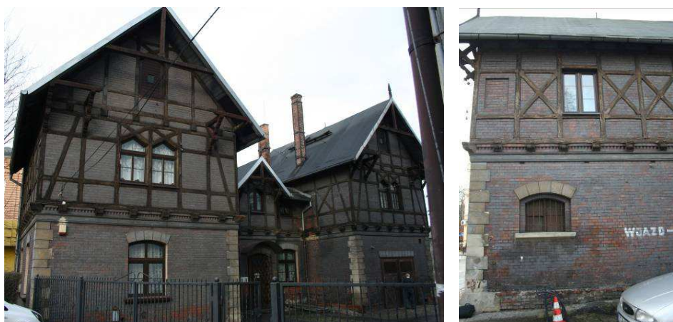
Fig. 3. Building of State Music School in Gliwice.
