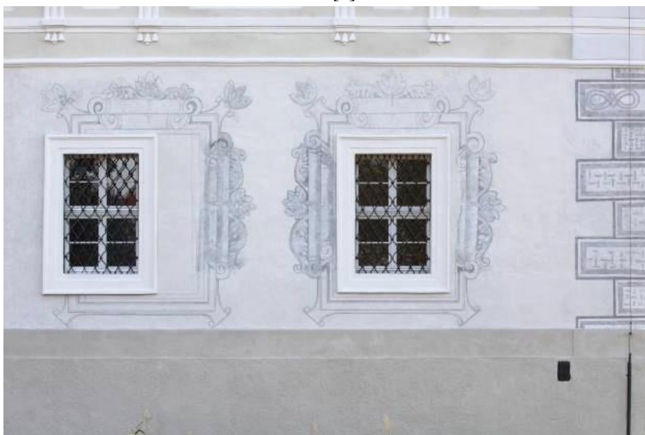
Fig. 2. Sgraffiti on the northern wall of the western wing of the palace in Zabór, after the work of conservation and restoration
