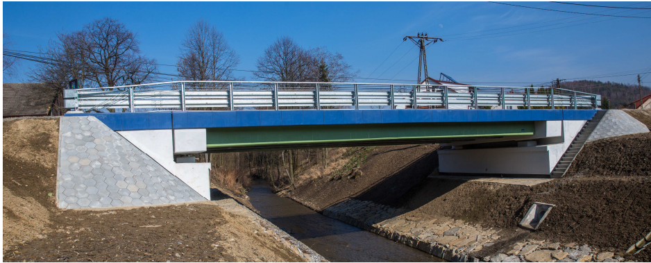
Fig. 8. Hybrid bridge made of FRP composite and concrete in Błażowa opened to traffic, Poland
