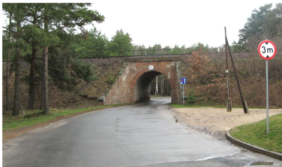
Fig. 1. General view of the railway viaduct
