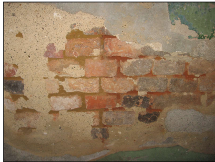
Fig. 4. Part of the western wall of the ground floor. Walls made of solid brick
