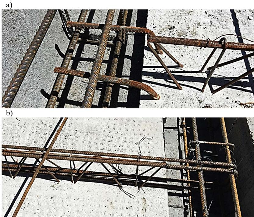
Fig. 6. Support reinforcement: a) rebars anchored from the top surface, b) U-type rebars
