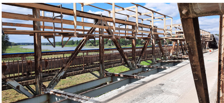
Photo 3. Renovation of the bridge steel structure
