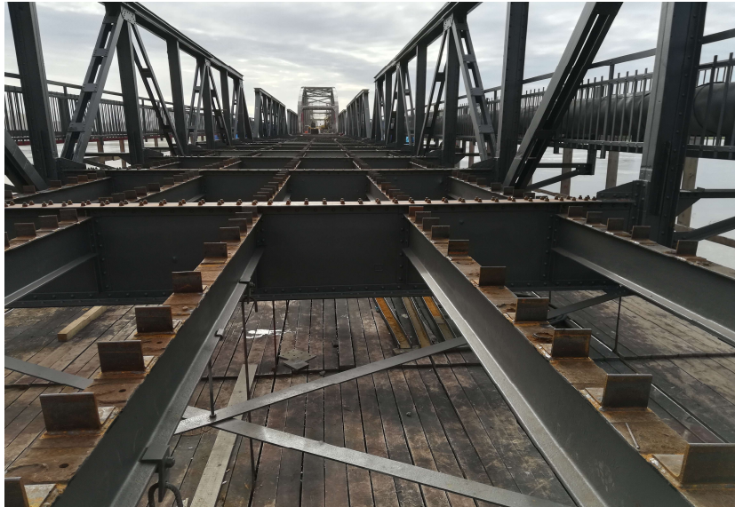
Photo 4. Replacement of the bridge slab
